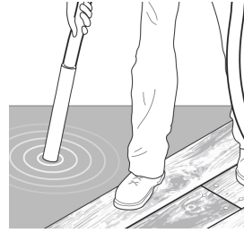
Vibrate concrete
